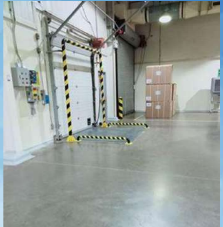
INSTALLATION OF EDGE BRUSH AND BUMP RAIL AT ESA BATANGAS
