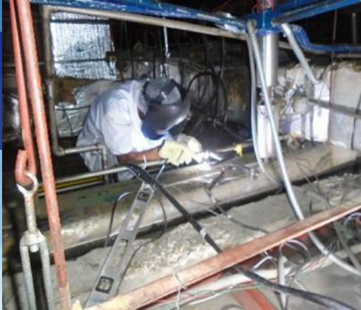
PROJECT PIA MODELEZ 2018: INSTALLATION OF 3PC VALVE DESIGN VALVE
