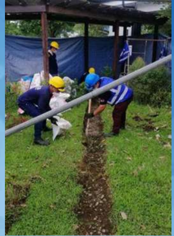
INSTALLATION OF DRAIN PIPE BATANGAS 2021
