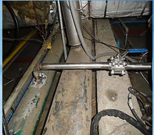
PROJECT PIA MODELEZ 2018: INSTALLATION OF 3PC VALVE DESIGN VALVE
