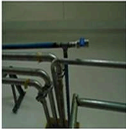
Compressed air connection with ss ball valve
