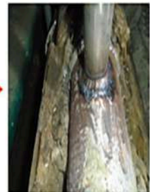
Steam line stub weld
