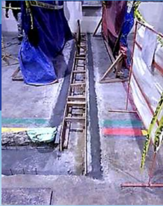
CONSTRUCTION OF CONCRETE TRENCH WITH STEEL GRATINGS AND CATCH BASIN WATER PROOFING ON WALLS MARIKINA 2019
