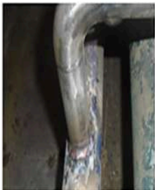
Compressed air line stub weld
