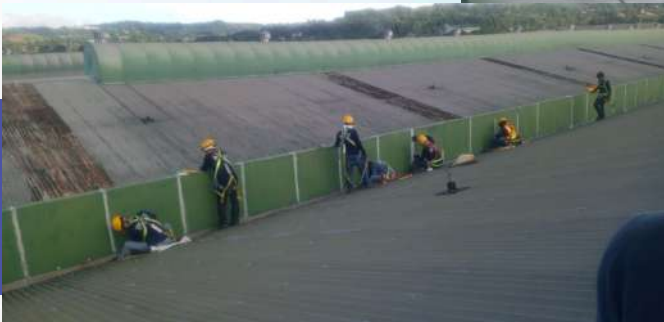
REPAIR OF LEAKS AT ANNEX ROOFING, PMFTC MARIKINA
