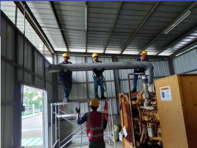
DISMANTLING WORKS: FDAS GENERATOR
