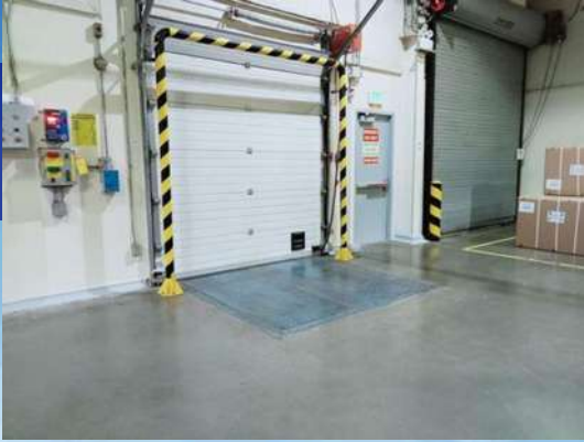
INSTALLATION OF EDGE BRUSH AND BUMP RAIL AT ESA BATANGAS
