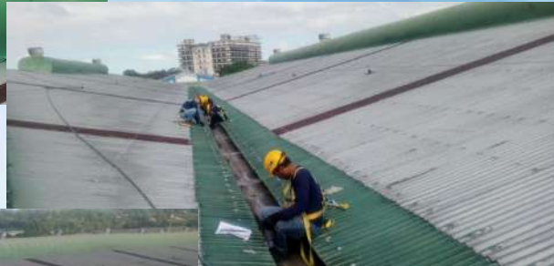
REPAIR OF LEAKS AT ANNEX ROOFING, PMFTC MARIKINA
