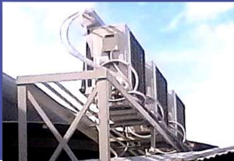
INSTALLATION OF 13 UNITS HYBRID AIRCON 2016
