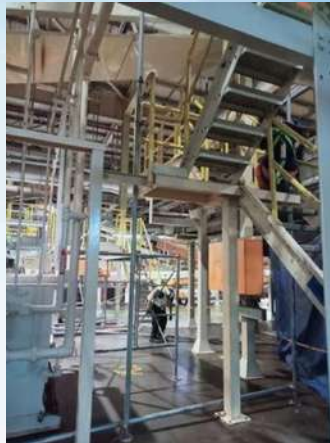
ERECTION OF SCAFFOLD, DISMANTLING OF CONVEYOR AT DCCC BATANGAS
