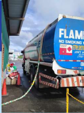
DE-WATERING OF CISTERN TANK AT WCL PMFTC BATANGAS PLANT
