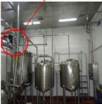
On-going tapping of steam line
